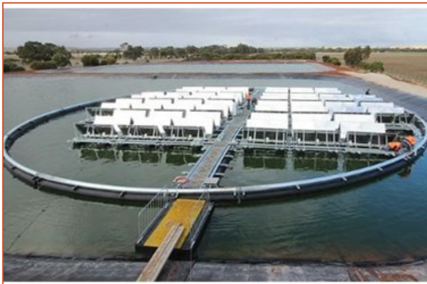
Floating solar system
