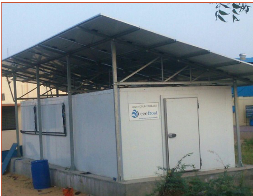
Solar-powered cold storage system
