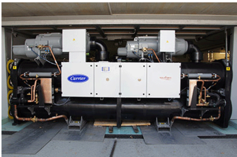
A Carrier Aquaforce chiller using R1234ze
