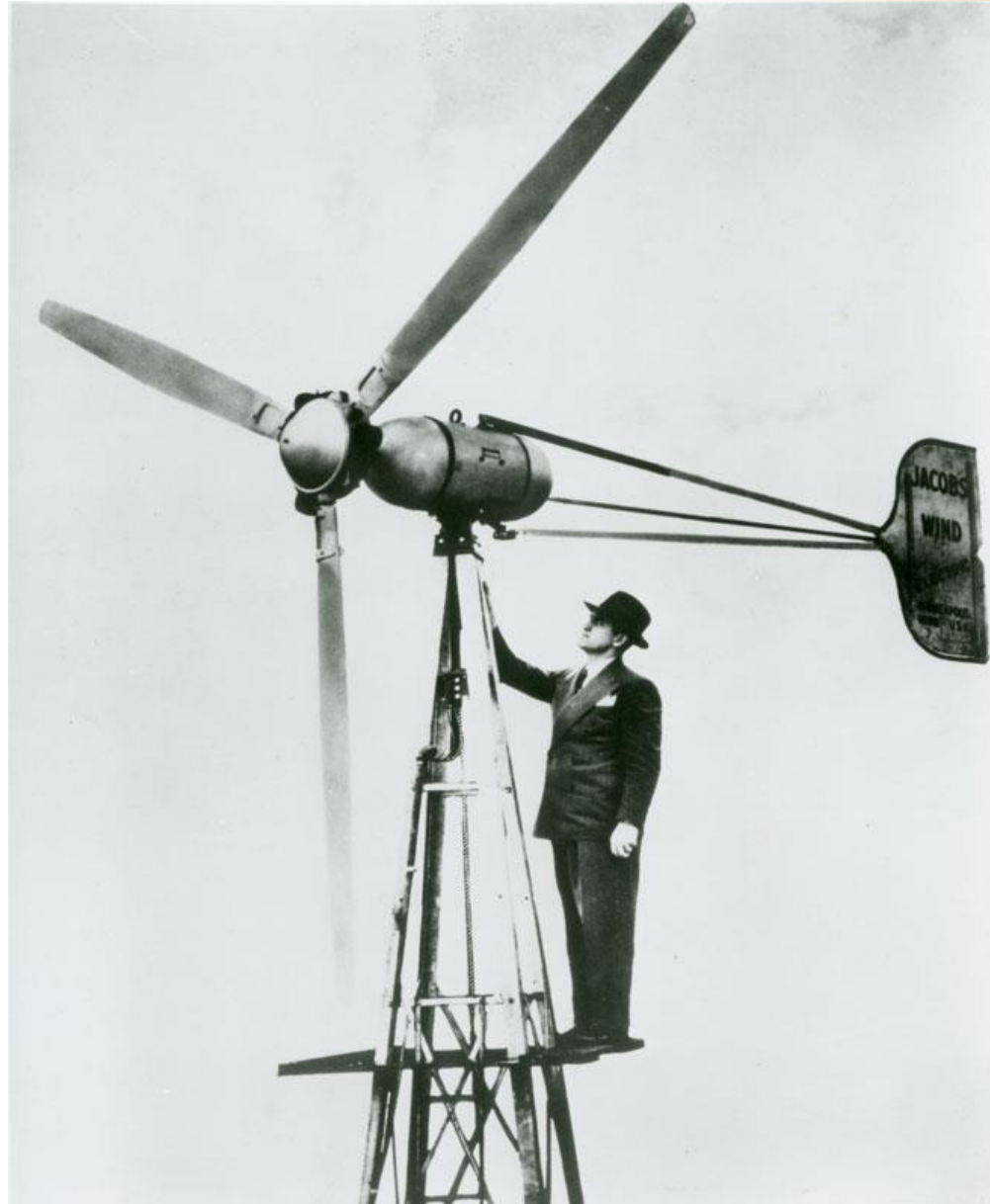
Jacob's 2.5 Kw wind turbine USA, circa 1940
