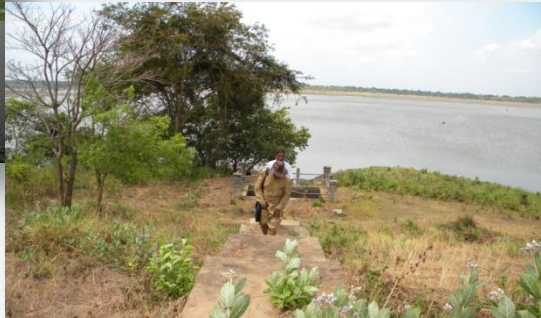
Middle level tanks
