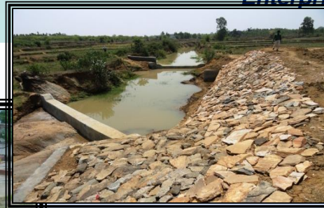
Check dams for ground water recharge in Koraput, Odisha.
