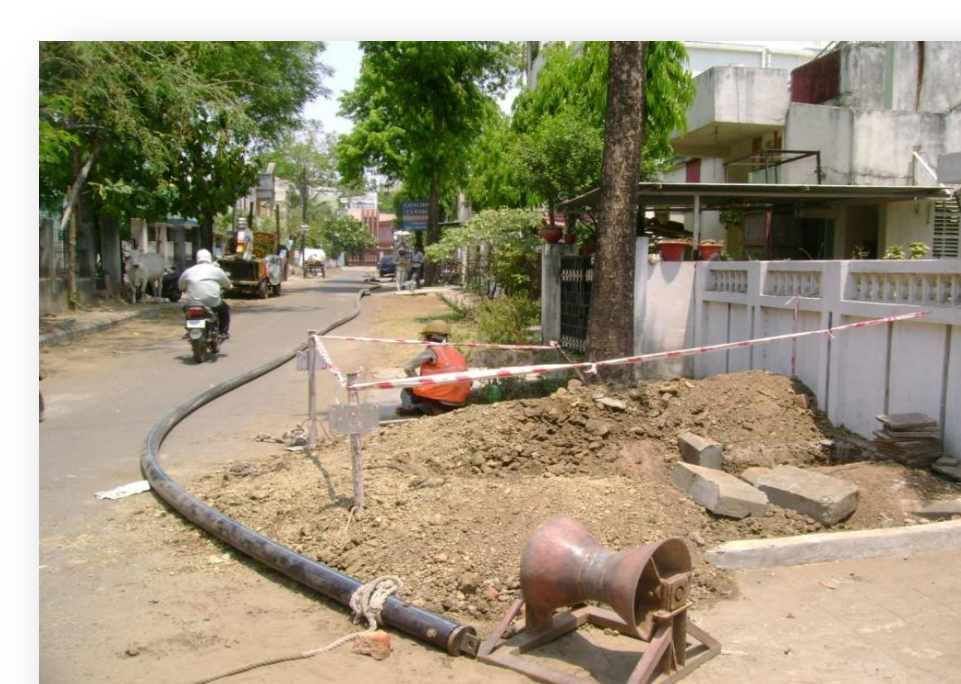
Laying of pipeline by Horizontal Directional Drilling (HDD)
