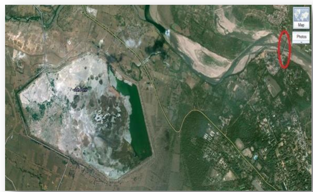
Ash pond in the catchment of Kanhan River
