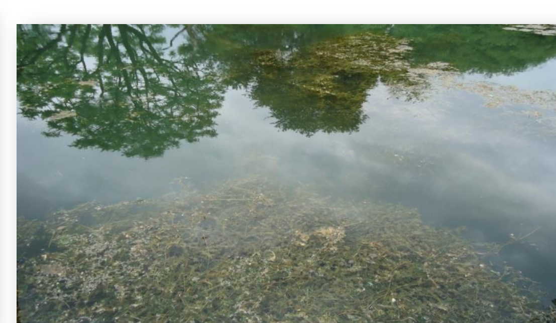
Aquatic Weeds in Clarifier at Old Gorewada Treatment Plant
