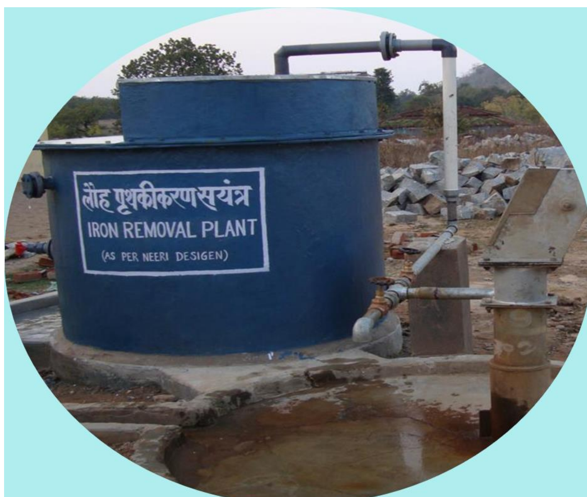
HP attachable Iron Removal Plant – FRP Structure (Can be fabricated in the factory and installed at the site in a few hours)
