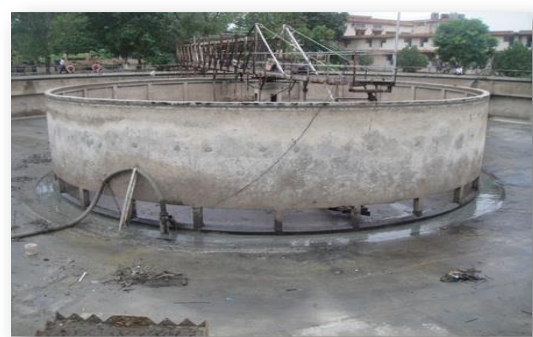
De sludging and repair of clariflocculators at Pench –II WTP
