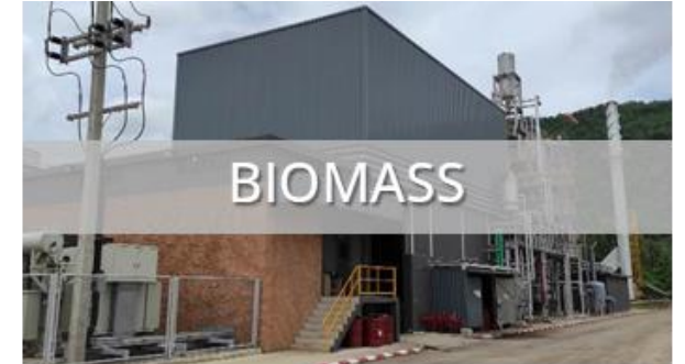
4.9 MW Biomass Power Plant @Ban Khao Noi, Phitsanulok
