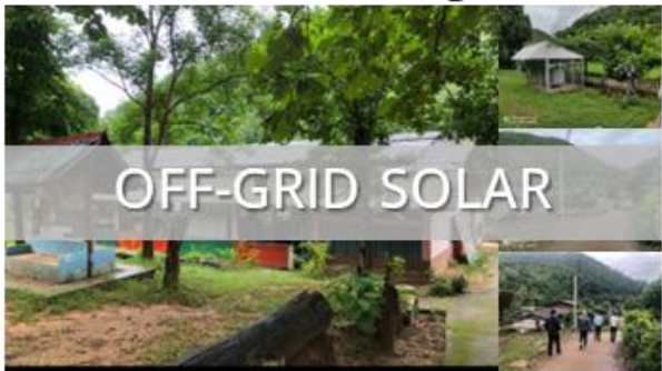
100 kW Microgrid @Ban Pha Dan, Lamphun
