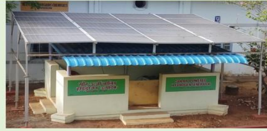
Solar Powered Hydrogen Generator (500 L/h)
