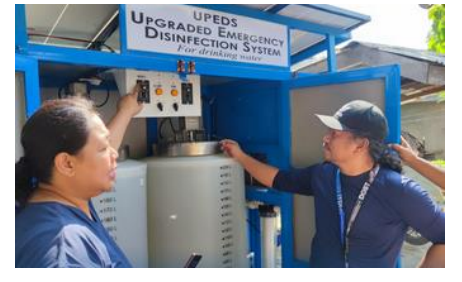
UpEDS Upgraded Emergency Disinfection System
