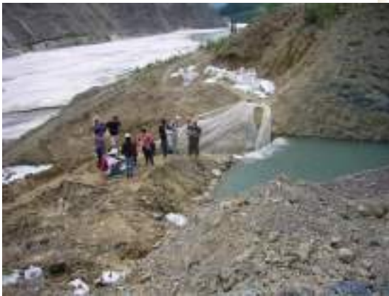
Tail water dam of Phosphate mining in Central Guizhou
