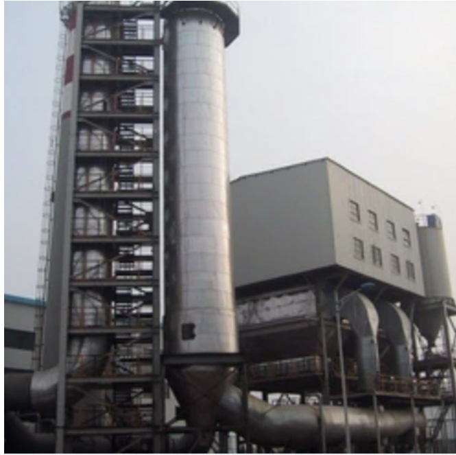
Figure 2.17 Evaporative gas cooling and conditioning (Source: https://www.durr.com/en/products/environmental-technology/exhaust-gas-and-air-pollution-control/sorpt-x-sorptive-processes/sorpt-x-ac ).
