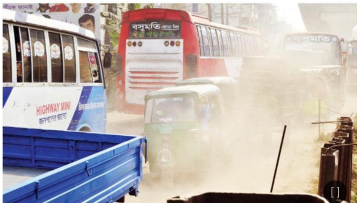
Figure 3.2.2: Severe dust pollution in construction sites
