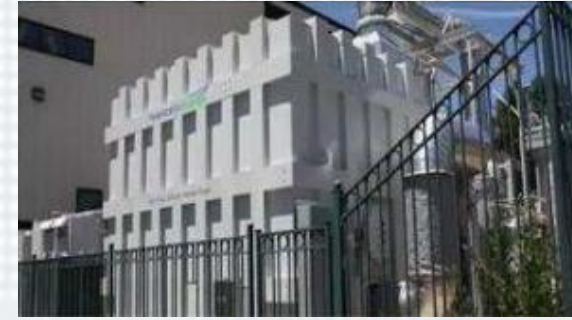
Solid oxide hydrogen production equipment
