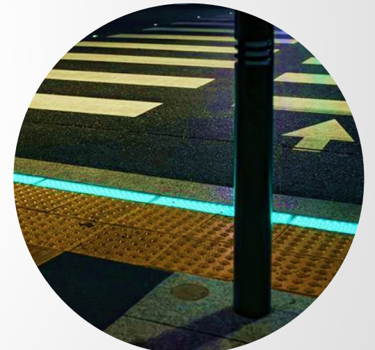
Crosswalk floor Traffic Light (Night)
