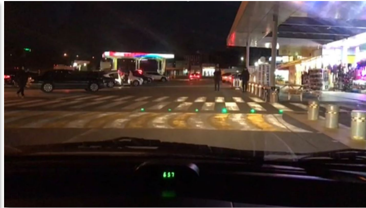
Energy Harvesting Road Installation at Manghyang Rest Area on Gyeongbu Main Highway
